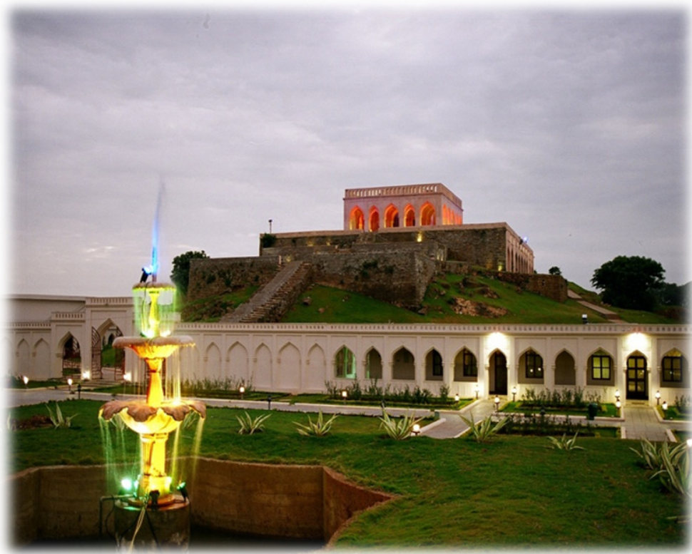
(Taramati Baradari Cultural Complex).
